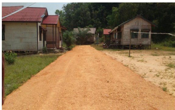
Completed road maintenance project at Tumbang Keminting village, Central Kalimantan.
