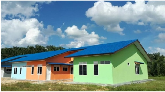
New housing provided for workers and their families at PT Agro Wana Lestari, March 2019.
