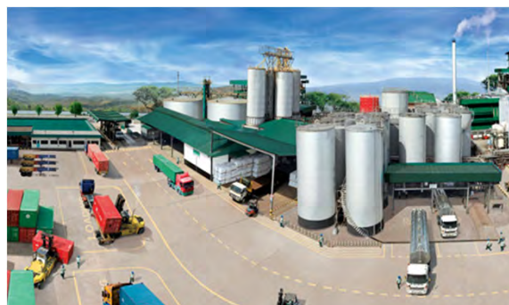
Refining facilities of Premium Vegetable Oils Sdn Bhd and Premium Fats Sdn Bhd, Pasir Gudang, Malaysia. The plants incorporate the capability for Palm Kernel Solvent Extraction and the production of specialty oils and fats
